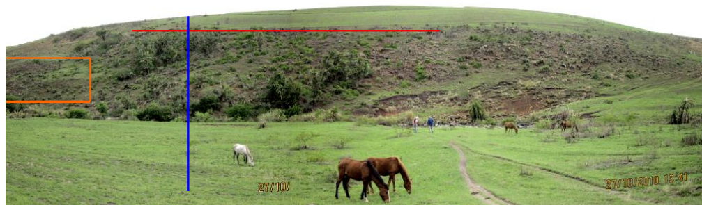
Plate 1. View of right flank. Red line indicates approximate upper dolerite contact. Blue line indicates previously drilled centre line. Orange rectangle indicates position of possible downstream quarry.
